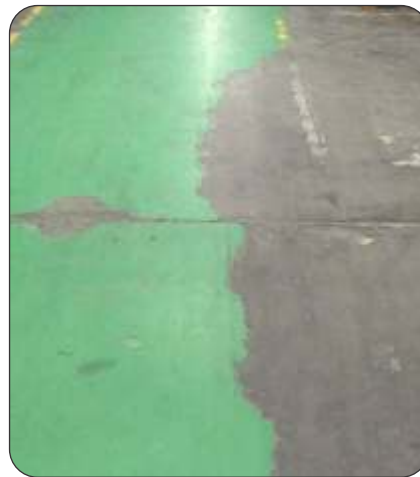
Eliminate Coating Failures
